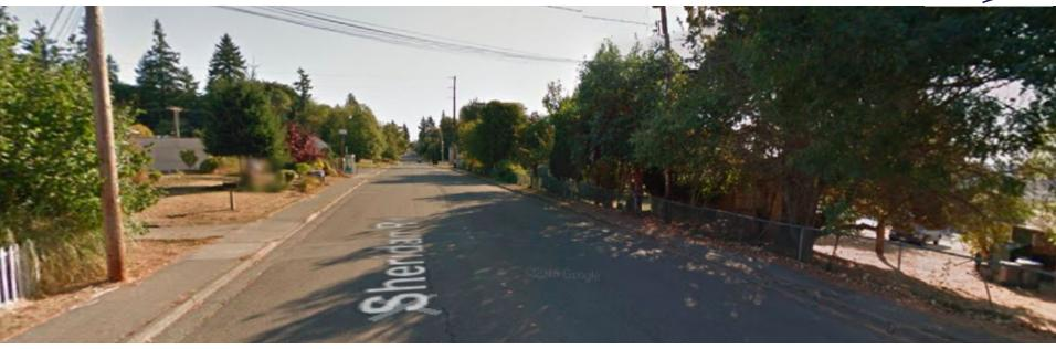
Note 34' roadbed without white fog lines along the entire length. Sidewalks are 5' on each side. Recent overlay leaves a 12" gap of old pavement at the curb, but the overlay is feathered and does not present a hazard. Note that there are several storm grates next to the curb on the north side.
