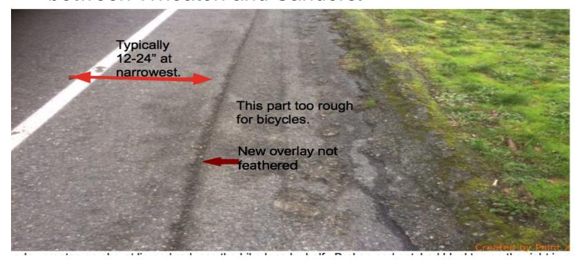
Recent overlay creates an abrupt lip and reduces the bike lane by half. Broken and patched blacktop on the right is not a safe riding surface. A smoothly feathered shoulder repaving of Sheridan's shoulders would make conditions much safer.
