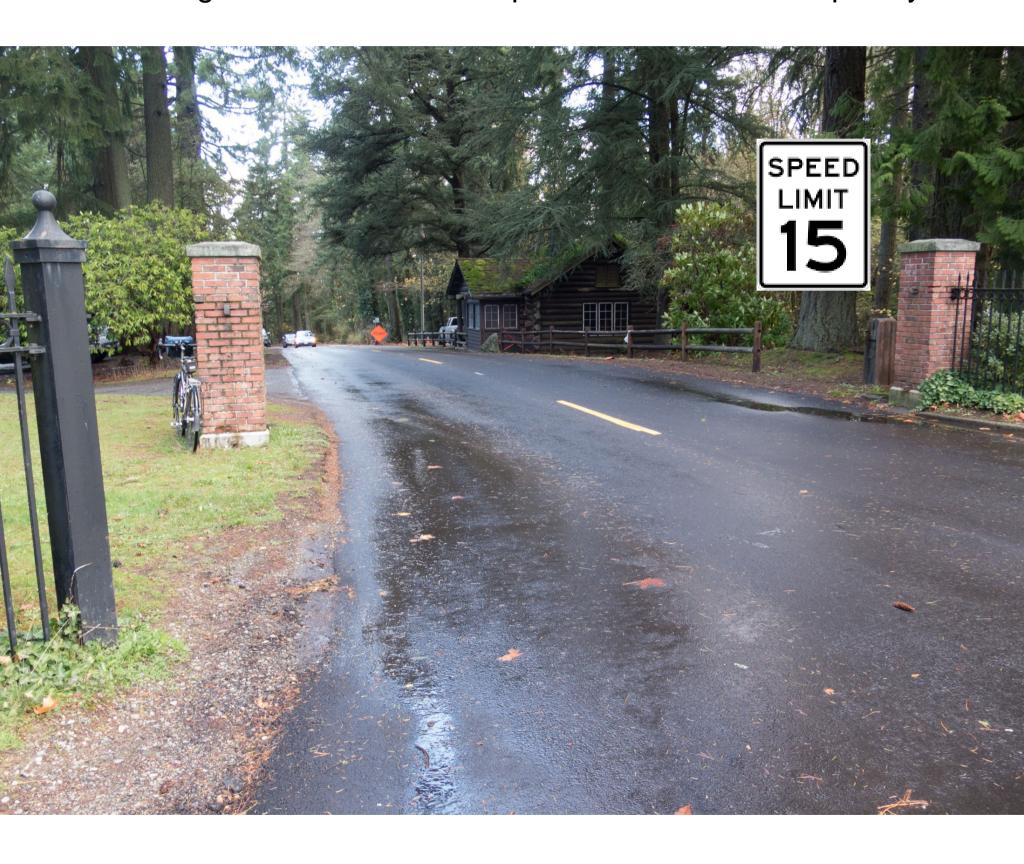
Available width varies from 23.5 ft at Cub Scout cabin to 26 ft. (Shoulder lane can be squeezed to 2.5 ft adjacent to cabin). Four feet is minimum width to officially mark a bike lane per MUTCD, so 3 feet shoulder markings should be used instead.
